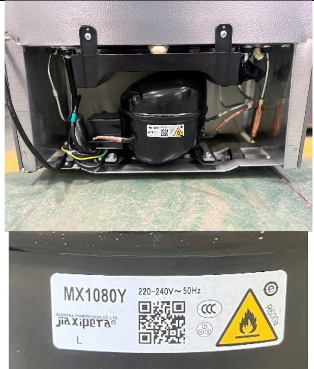
Picture 4 Compressor chamber, Picture 5 compressor
